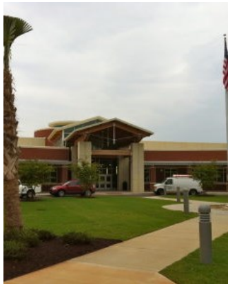
River Bluff High School Front Entrance
